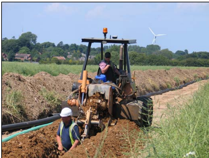
Figure 6 The on site laying of the underground cable
