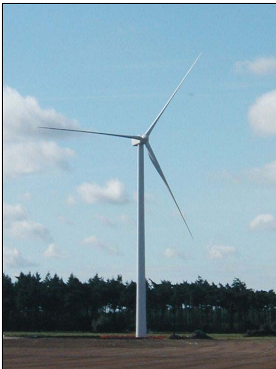
Figure 3 A typical turbine unit
