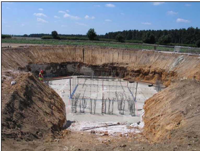
Figure 4 Excavating for a foundation
